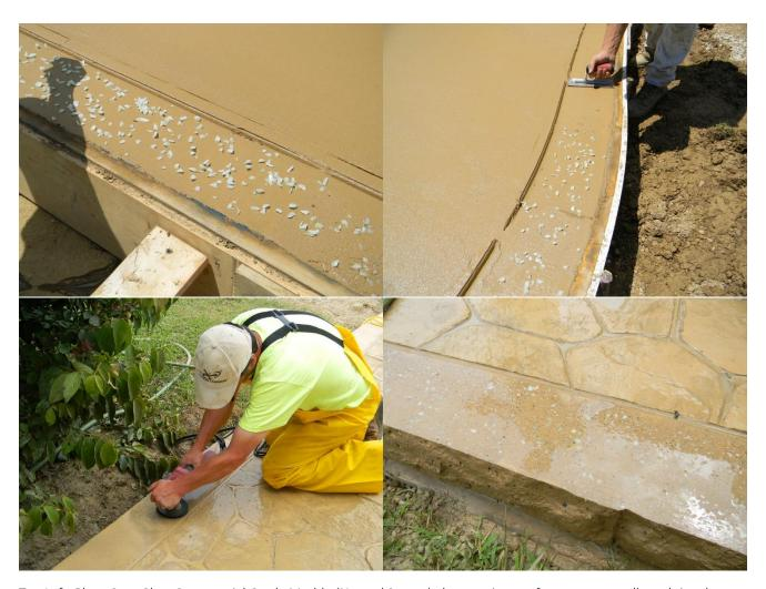
Top Left: Place Core Glow Commercial Grade Marble (Natural Stones) along project surface area once allotted time has passed. Surface should be stiff but not hard. Top Right: Press stones into the cement surface. Bottom Left: Sand down surface area once cement has set. Bottom Right: Finished concrete surface with glow stones embedded permanently in the surface.
